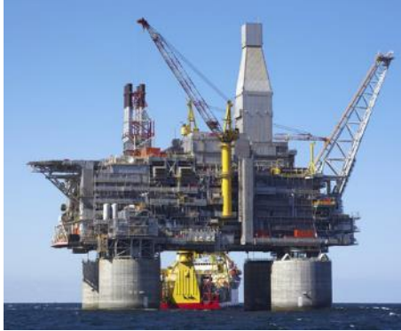
Energy / Oil & gas
